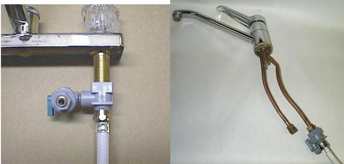
The EZ Faucet Connector Valve gives you a quick, easy and reliable water supply for your water filter. It provides full flow – great for homes with low water pressure. It's easy to install:
